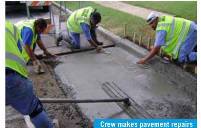
Crew makes pavement repairs
