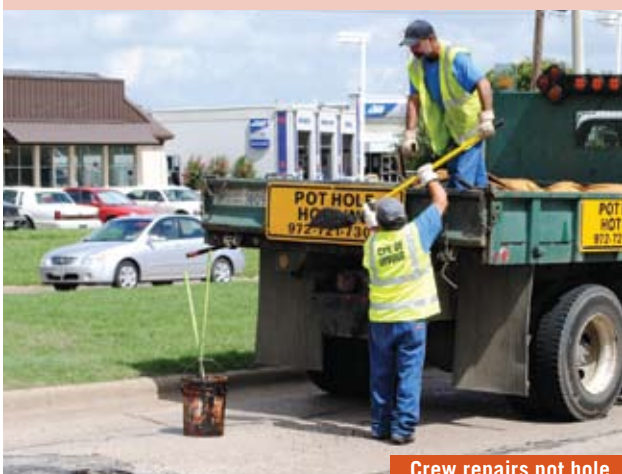
Crew repairs pot hole
